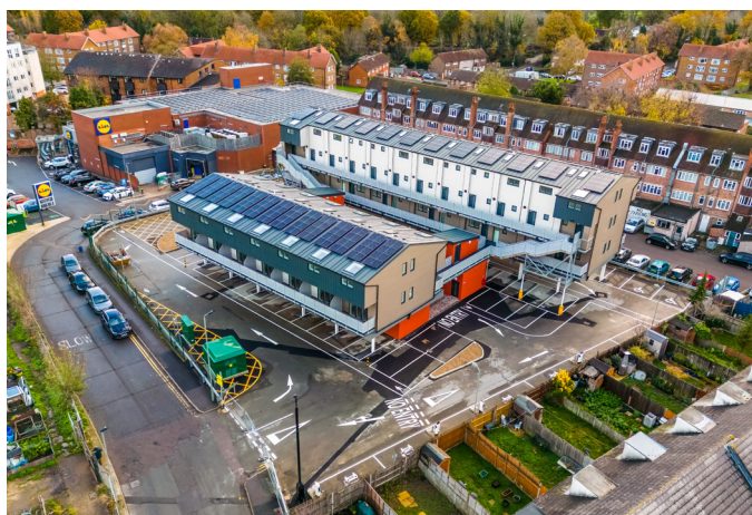
Above: On-site Construction — minimising on-site works reduce the amount of noise pollution generated by machinery for cutting, drilling; fitting out the modules off-site means that for less materials and components are stored on site helping to keep the area clean and tidy; Off-site material cutting and processes reduce amount of airborne dust created during works, improving air quality.
