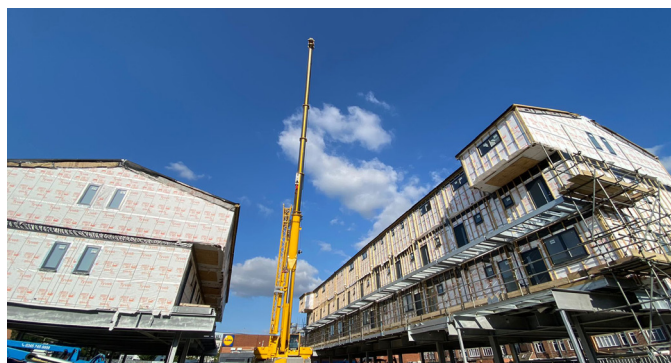
Above: On-site Construction — minimising on-site works reduce the amount of noise pollution generated by machinery for cutting, drilling; fitting out the modules off-site means that for less materials and components are stored on site helping to keep the area clean and tidy; Off-site material cutting and processes reduce amount of airborne dust created during works, improving air quality.
