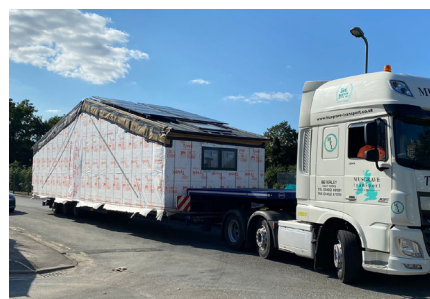
Above: Off-site Production — up to 90% of the building work is completed in the UK based factory so once the groundworks are completed, the units were delivered to site and installed in matter of weeks.
