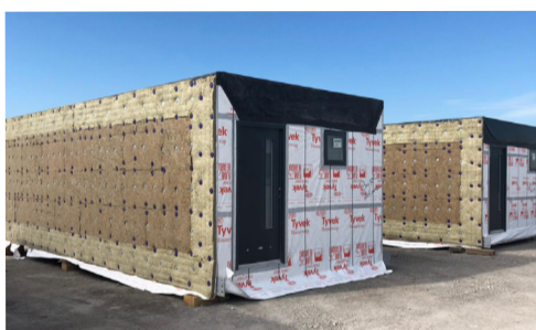
Above: Off-site Production — up to 90% of the building work is completed in the UK based factory so once the groundworks are completed, the units were delivered to site and installed in matter of weeks.
