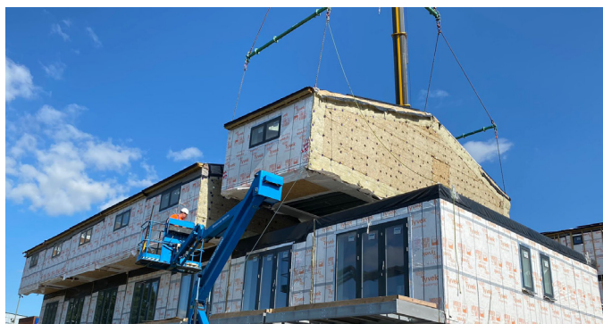
Above: On-site Construction — minimising on-site works reduce the amount of noise pollution generated by machinery for cutting, drilling; fitting out the modules off-site means that for less materials and components are stored on site helping to keep the area clean and tidy; Off-site material cutting and processes reduce amount of airborne dust created during works, improving air quality.
