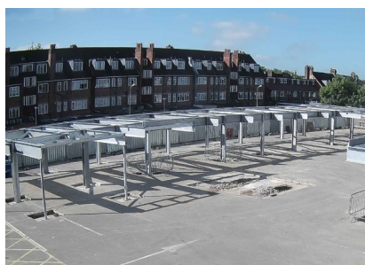
Above: The steel podium platform be installed in days than months
