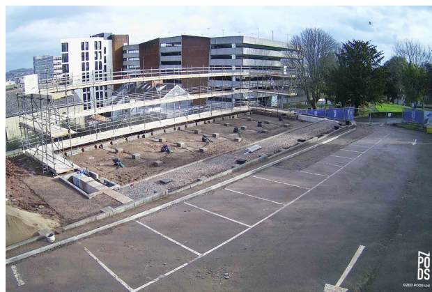
Groundwork completed on site ready for module installation
