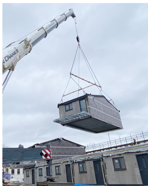
Housing modules manufactured in UK factory
